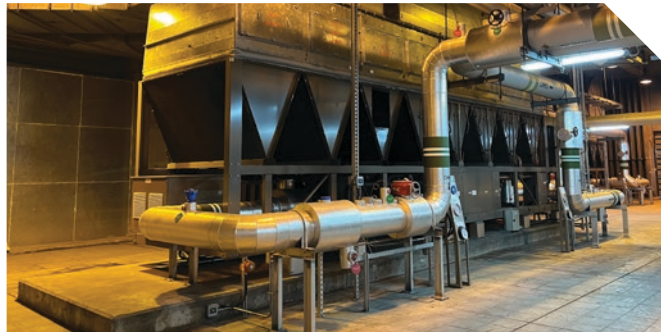
Large-scale chiller replacement project
